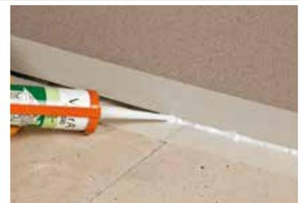
Expansion joints should have minimum width of 6-10 mm. Expansion joints should be insulated by using proper profiles or mastics. Cementitious grouting materials are not appropriate for expansion joints.
