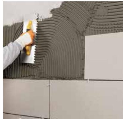
According to the size of the tiles, fix tiles with either single buttering method (the adhesive is buttered on the substrate) or double buttering method (for tile sizes > 33x33 cm, adhesive should be buttered onto the tile back as well). The tiles must be fixed within the open time of adhesive and pressed on with a twisting and sliding action to achieve a good contact.
