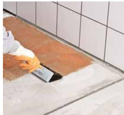
■ When tiling onto substrates with low porosity (water absorption rate < 3%), high performance adhesive should be chosen.
