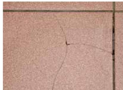
The grouting materials filled into joints should be flexible sufficient to absorb the movements occurring in horizontal with the surface. Too stiff grouting materials will fracture or depart from the tiles' edges.
