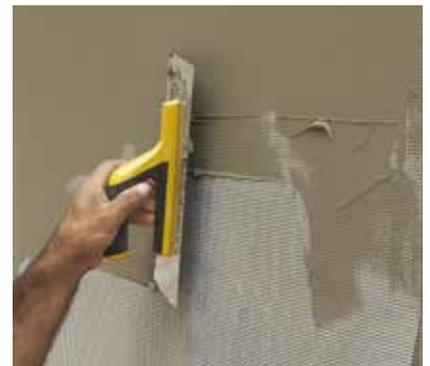
■ Adhesion and rigidity of the existing tile covering should be checked by tapping a hammer. Loose or poorly adhering covering should be removed and replaced by similar covering or the substrate should be reconstituted with a suitable repairing product. Before plastering onto existing tiles, surface adhesion should be improved for impervious the substrate with primers including thick fillings.
