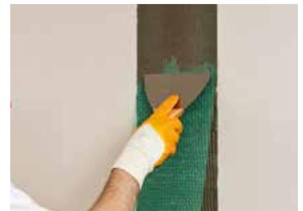
As a preparation to paint coating, the substrate should be plastered with two coats;
