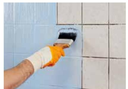
When tiling during hot, windy and dry conditions, it is inevitable that the mortar will lose its mixing water very fast due to rapid evaporation. Prior to spreading the mortar on the substrate, wetting or damping will decrease substrate surface temperature reasonably. For better performance, the surface should be sealed with appropriate primers.
